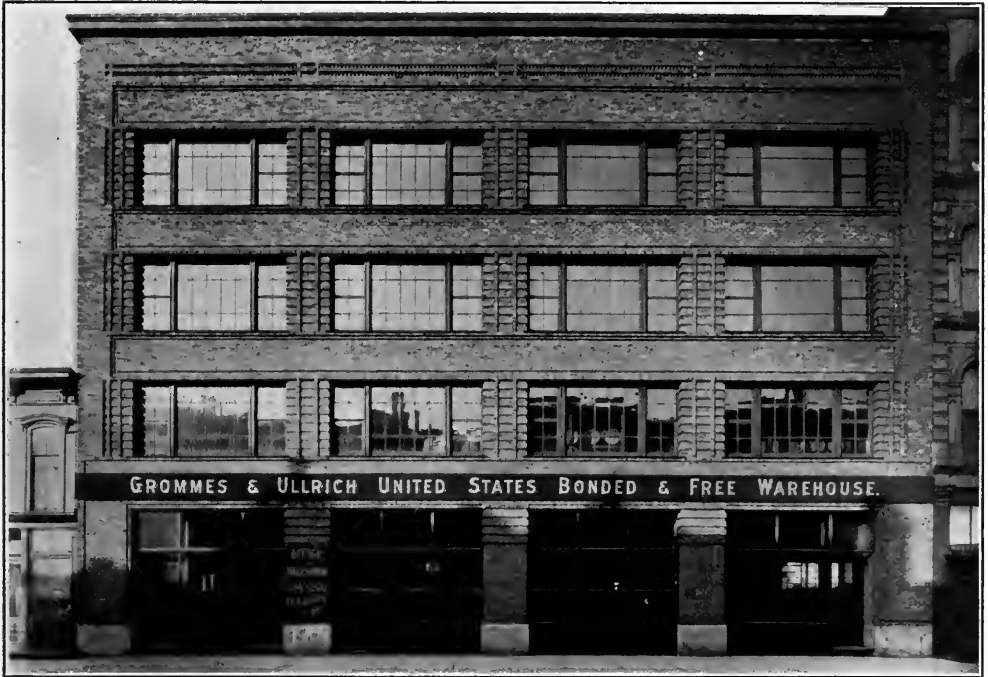
FIG. 3.—A WAREHOUSE IN CHICAGO.
